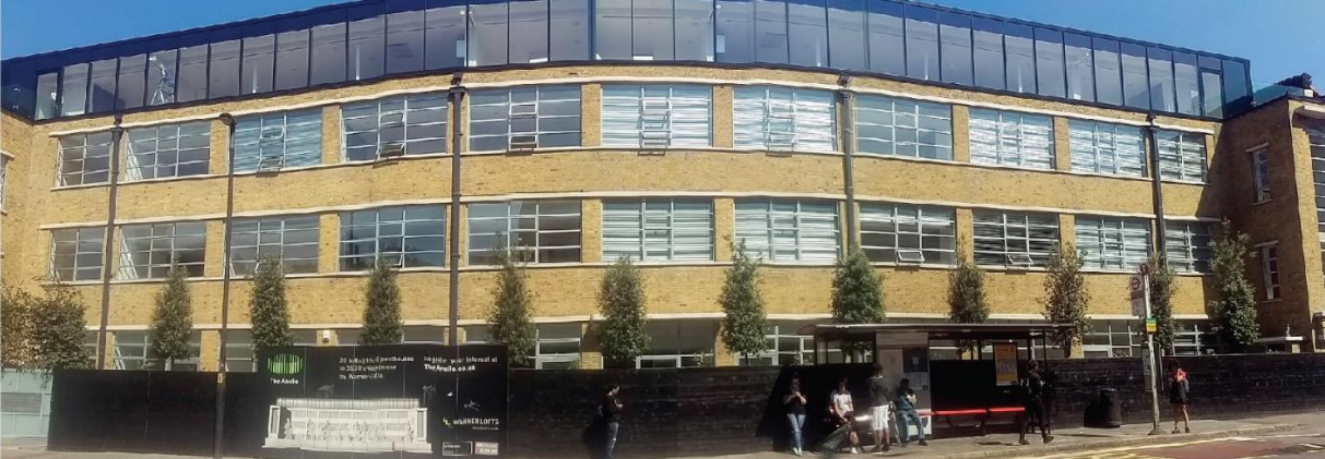
Figure 1. South-West facing building close to Camden High Street Underground Station (Photograph taken with a wide-angled lens).
